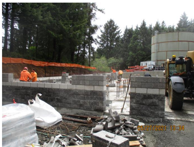
Beaver Creek Intake Pump Station Building and CMU Construction:
