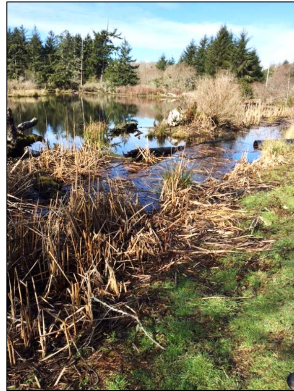
Photo 14. Proposed backwash outfall site at right bank of Beaver Creek. Looking south from right bank. Looking southwest from North Beaver Creek Road.
