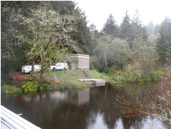
View of intake from South Beaver Creek Bridge:
