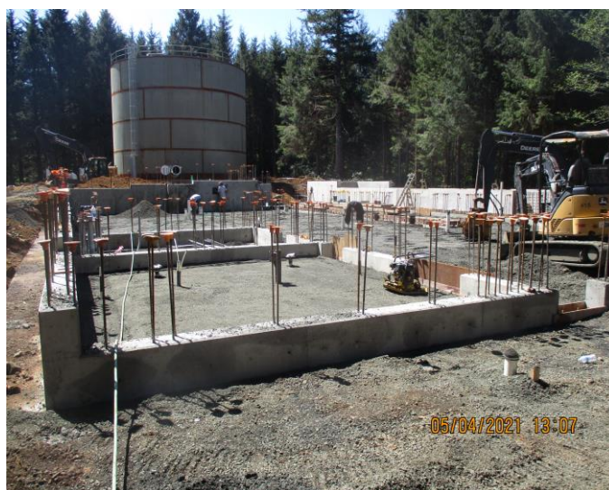
Membrane Building Construction with Clearwell in the background and Backwash Basin to the left:
