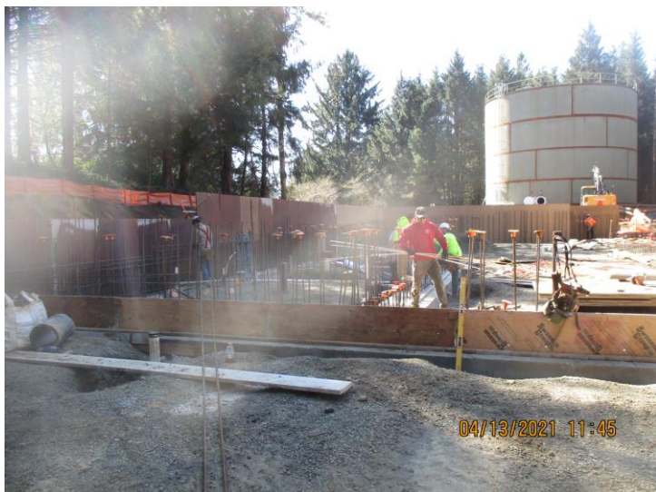
Membrane Building Construction with Clearwell in the background and Backwash Basin to the left:
