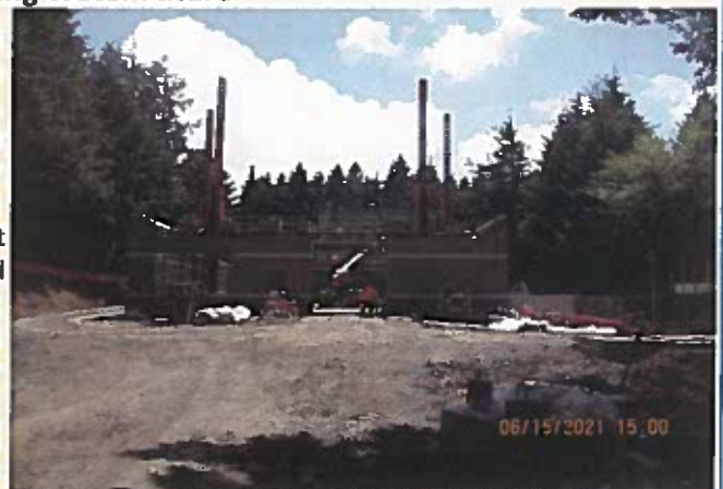
SRWD Membrane Treatment Building Under Construction
