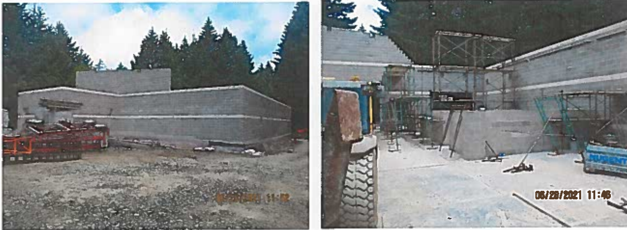
Membrane Building Block Wall Construction:
