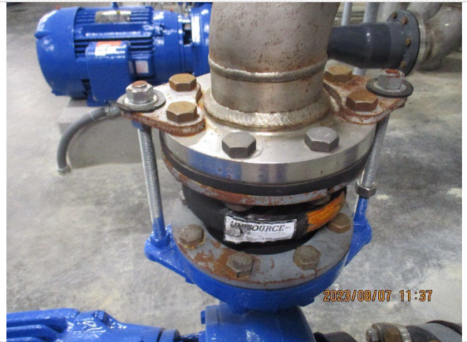
Rusting on bolts observed at FW pumps
