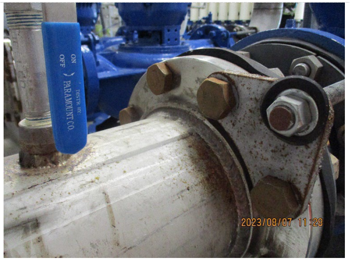
Rusting on bolts observed at FW pumps
