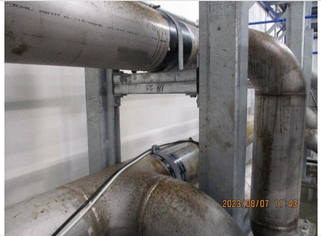
Leak at the joint of the CIP pipe
