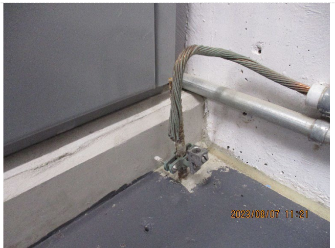
Ground to structural not connected and corrosion observed. This is a code violation.
