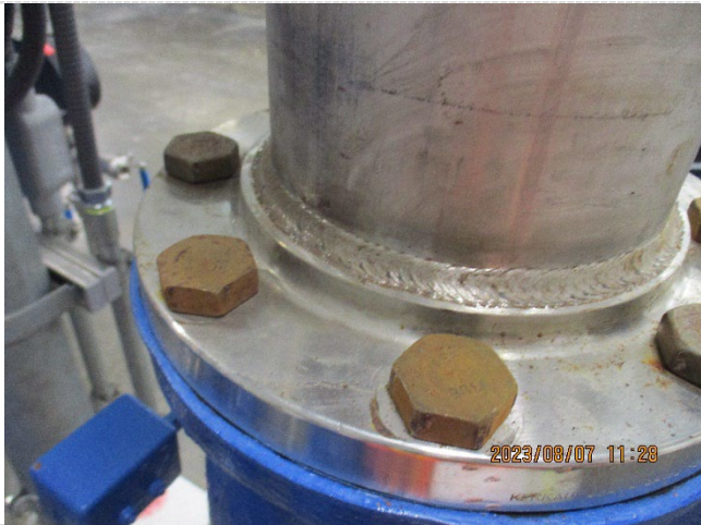
Rusting on bolts observed at FW pumps
