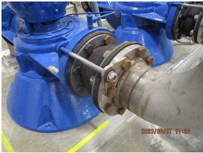
Rusting on bolts observed at FW pumps
