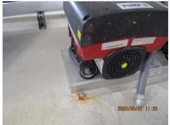
Ground to structural not connected and corrosion observed. This is a code violation.
