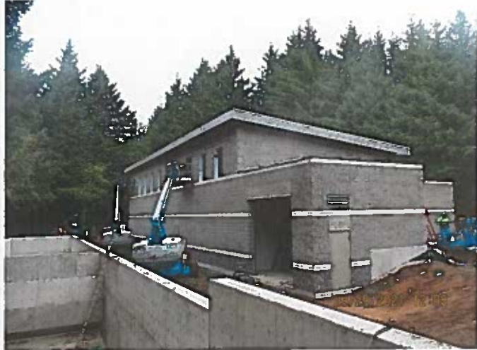
WTP window installation:
