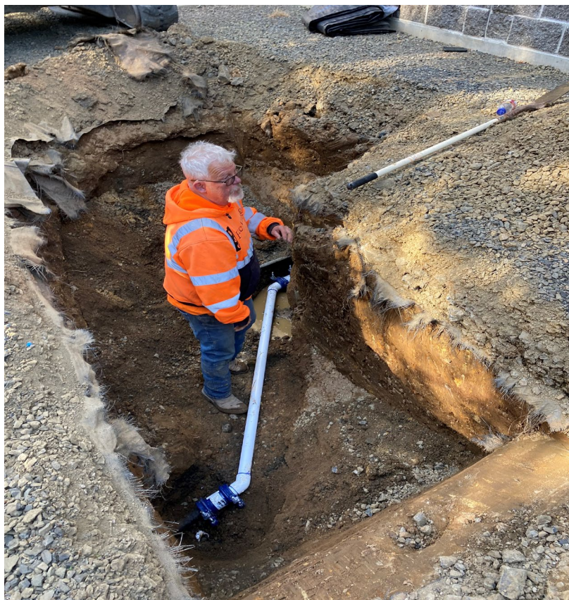
2-inch Drain Line Repair:
