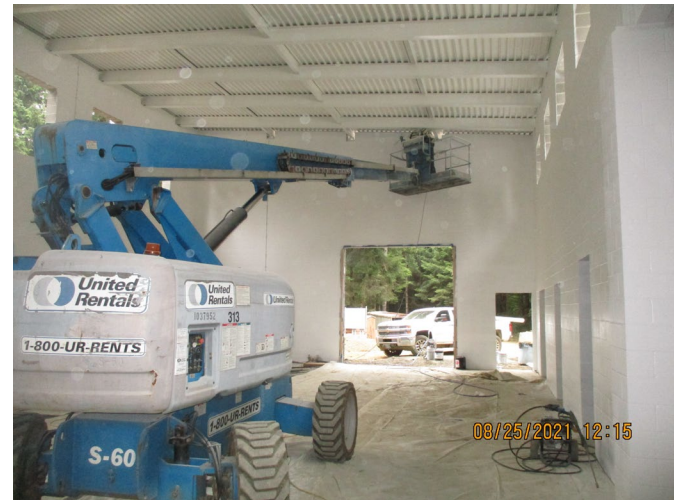
Interior painting Membrane Building:
