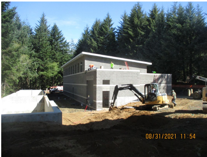
Completed Backwash Basin:
