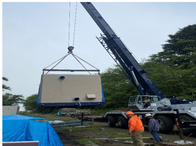
123 rd Street Pump Station:
