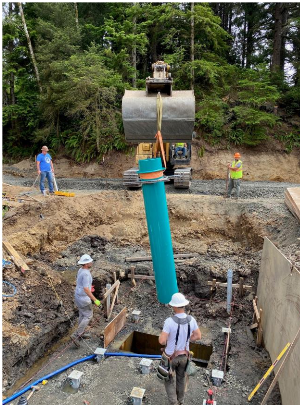
Beaver Creek intake piling installation and pump can installation August 3, 2020:
