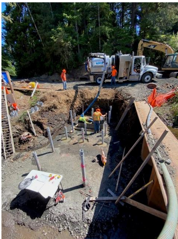
Beaver Creek intake piling installation and pump can installation August 3, 2020:
