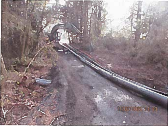
Pipeline placement towards Kona Place
