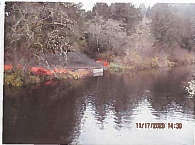
RW intake structure and surcharge loading – no activity in the month of November other than reestablishing BMPs
