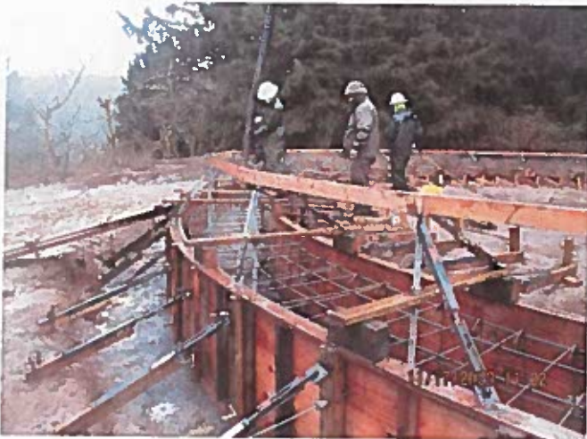
R&G concrete crew working on concrete pour for ringwall footing
