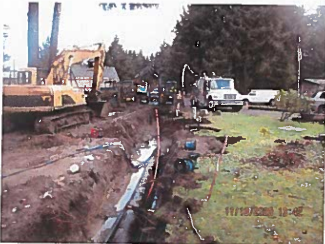
Contractor continues to install pipeline up to Kona
