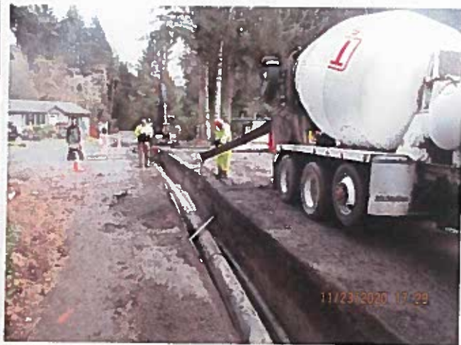
CLSM placement in pipeline trench at Kona Place
