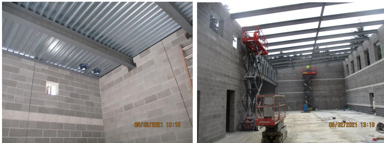
Membrane Building Construction:
