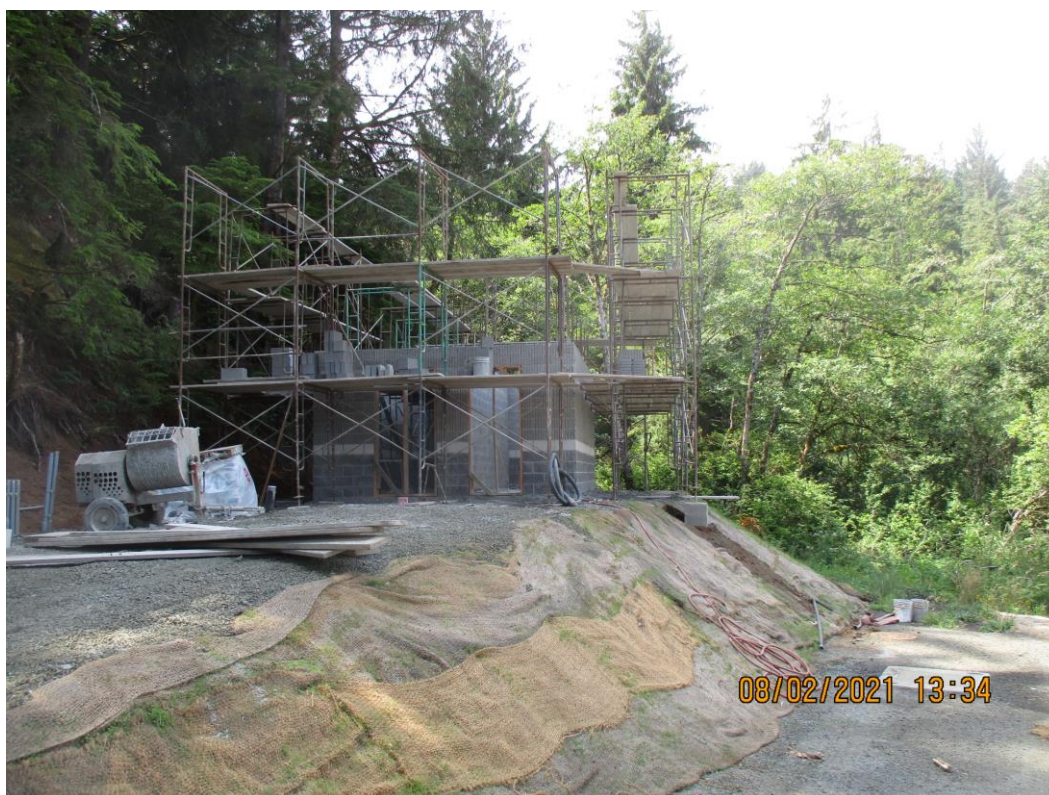
Beaver Creek Intake Pump Station Building and CMU Construction:
