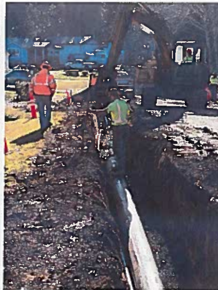
Kona Street pipeline installation:
