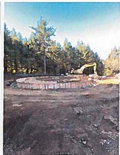
Clearwell ringwall forms:
