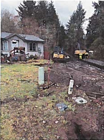
Pipeline into Makai Community:
