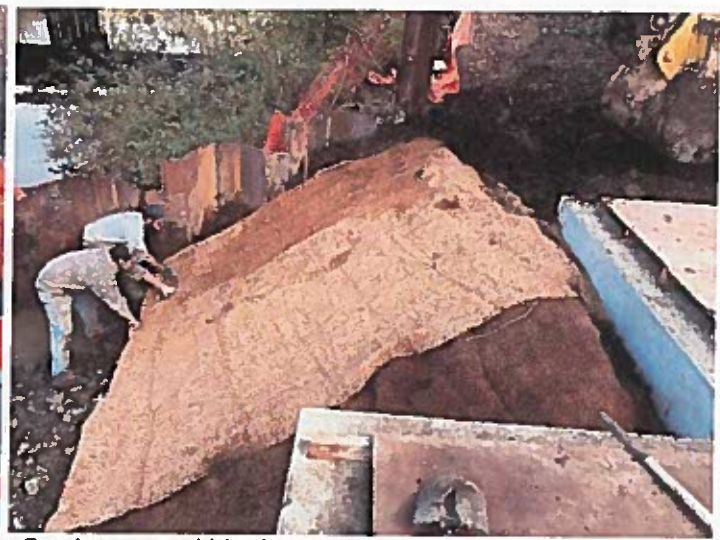
Erosion control blanket in front of the intake:
