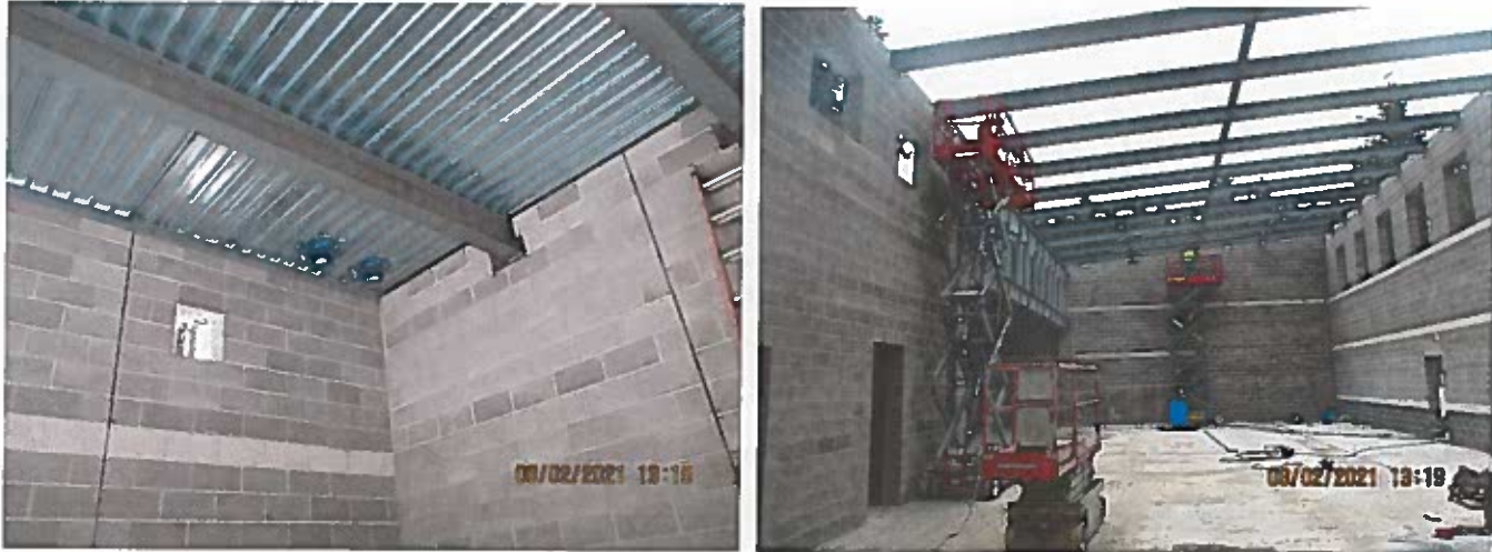
Membrane Building Construction:
